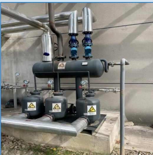
Condensate harvesting system at SHPL
